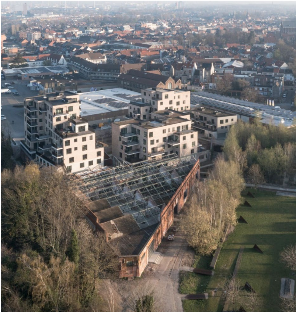
Figure 4.40 Cohousing Bijgaardehof also has a transition zone towards the neighborhood park. Between the walls of a former factory, the community shares a vegetable garden with the higher socio-spatial scale of the neighborhood.
