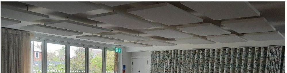
Figure 4.83 Also Cohousing New Ground had to install acoustic panels to make the common living room usable by more than a handful of people.
