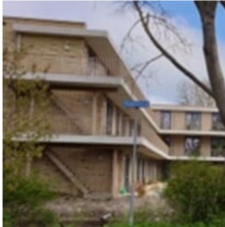
Figure 4.29 At Knarrenhof Gouda each level has a setback providing more daylight to the floors below.
