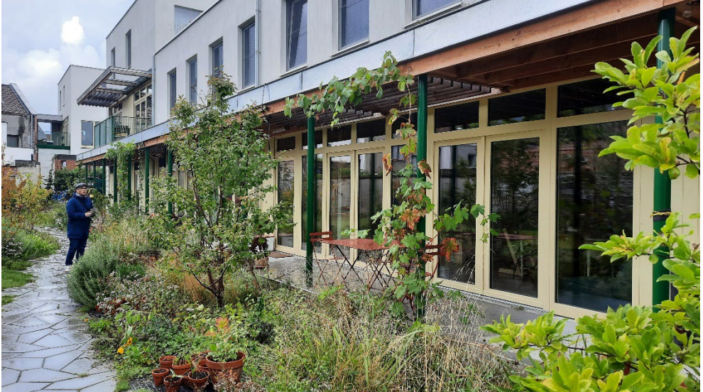
Figure 4.27 At Cohousing JEAN the scale level of the household has a little terrace and high greenery to the path that is used by the community of 10 households. Residents stated that despite the large windows, they usually keep their curtains open which is rare in Belgium. Note that this is not a public street. The size and effectiveness of a transition zone very much depend on how big the transition is between socio-spatial scales.
