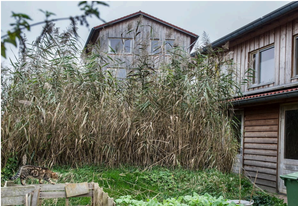
Figure 4.135 At Strowijk IEWAN in Nijmegen, residents allocated a part of their shared outdoor space for a constructed wetland to filter “grey” waste water.
