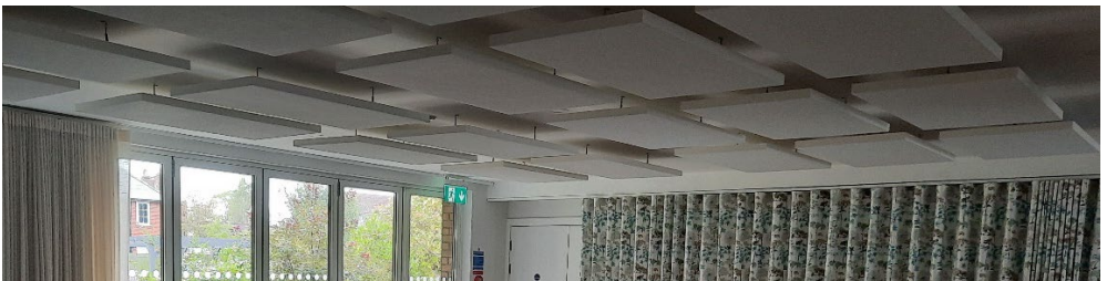
Figure 4.83 Cohousing New Ground also had to install acoustic panels to make the common living room usable by more than a handful of people.
