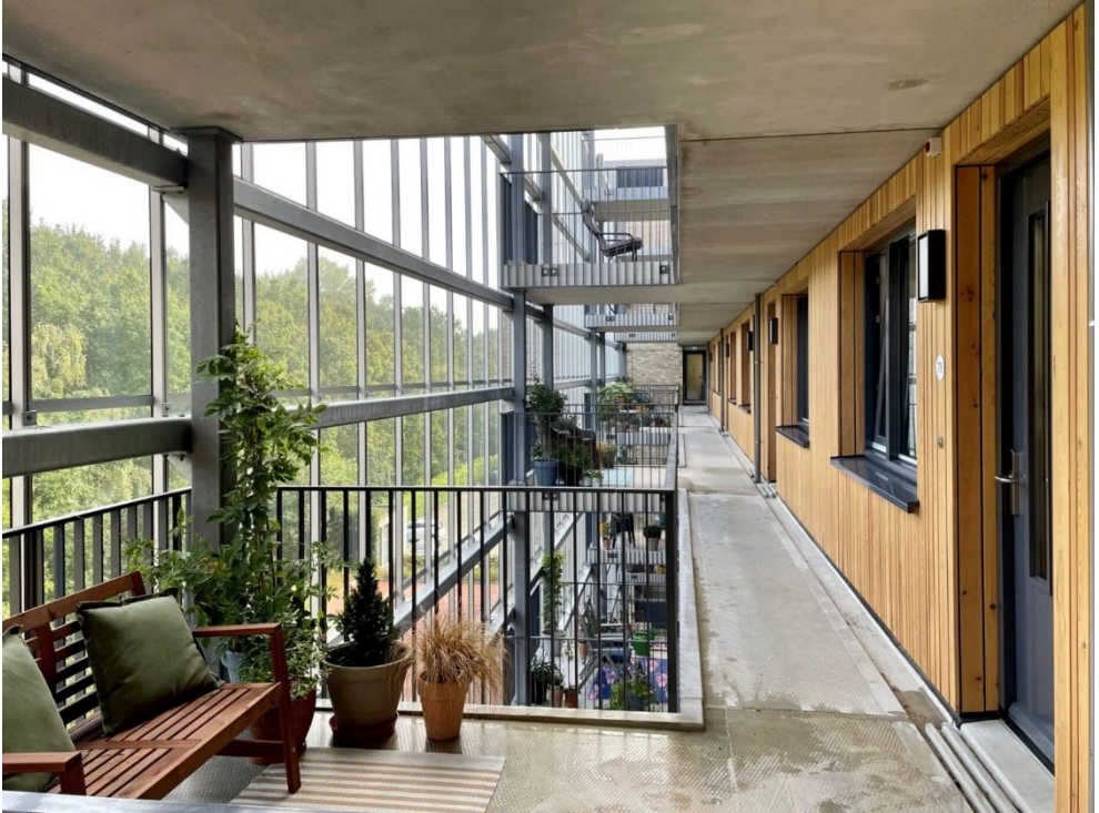
Figure 4.31 A walkway variant where the private balconies stick out is a common solution. However, here the private areas do no longer serve as transition zones between the walkway and the windows. Another disadvantage of this model is that the private areas are surrounded by more public spaces. Here the transition zone does not offer refuge anywhere (Browning et al, 2014). Refuge is the feeling of safety that a wall at your back provides.
