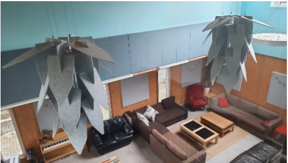
Figure 4.82 Cohousing Marmalade Lane, like many other communities, struggle with acoustics in their shared spaces. They had to install expensive acoustic panels and chandeliers to dampen sound to make the spaces more usable.
