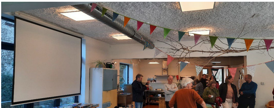
Figure 4.85 The acoustics ceilings of shared spaces in Cohousing Bijgaardehof.
