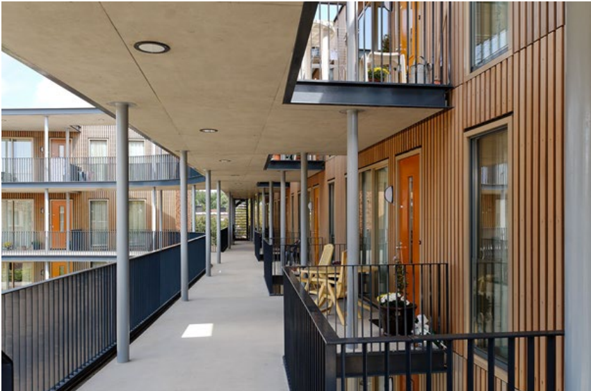
Figure 4.30 There are also various forms of walkways away from the windows with balconies.
