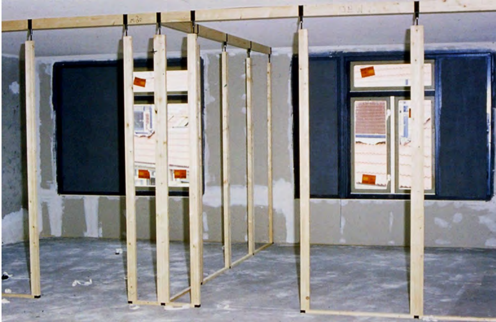
Figure 4.142 Flexible walls were at the core of the design of Gemeenschappelijk Wonen Nieuwegein by architect Flip Krabbendam. In 2010 a big renovation removed the flexible walls because of their bad sound insulation (Krabbendam, 2020).
